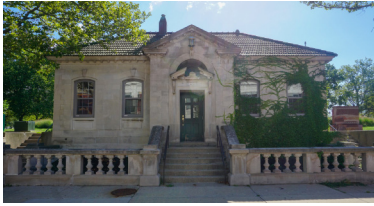
4. Veterans Park building renovations
